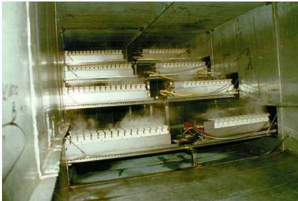
Example for a assembly of ENS-humidifier
